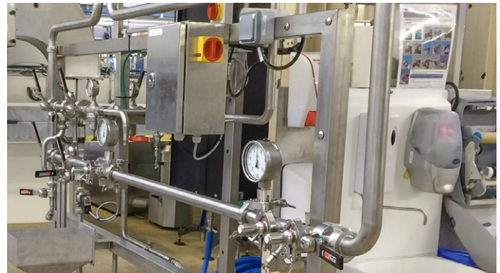
Figure 5A: Process Flow With Spacer Installed
