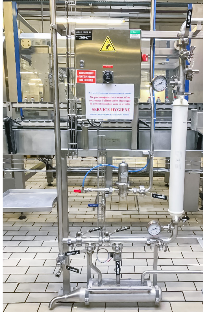
Figure 8: Capsule Filter Vertical Installation at POU
