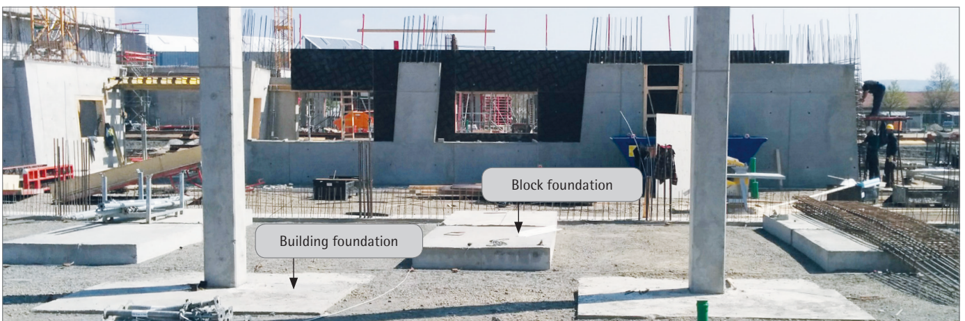
The building foundations and the block foundations for the anti-vibration weighing tables used for calibration were separately cast.
