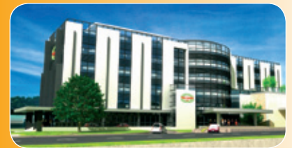
The Tien Phong Plastic JSC company building
