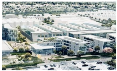
Goettingen, Germany Extension of headquarters
