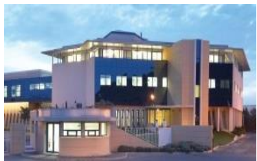
Aubagne, France Capacity extension of bag production
